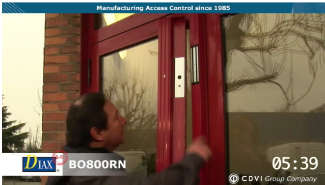
5 - Align the armature handle
