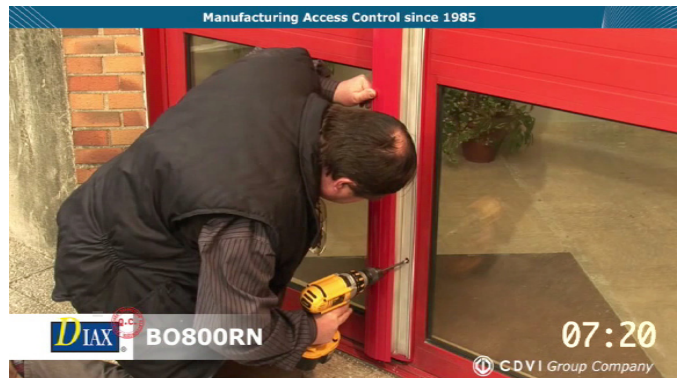
6 - Drill and fix the armature handle
