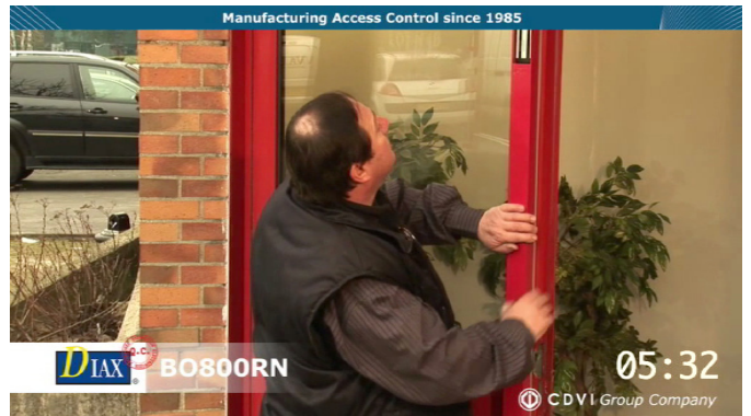
4 - Snap on the magnet housing cover
