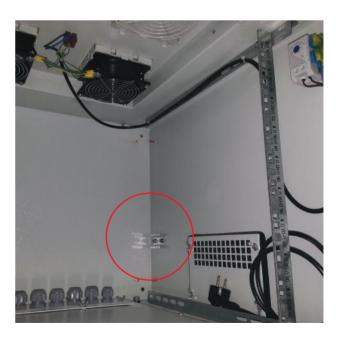
The assembly rail of the panel heater (at the lower rear right corner of the cabinet)  $\,$
