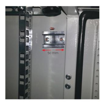
Assembly rail of the thermostat (at the upper front right corner of the cabinet)  $\,$
